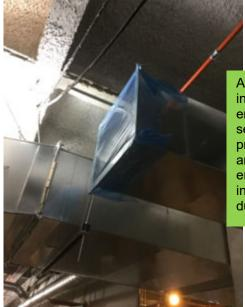
After installation, ends are still sealed to prevent dust and dirt from entering interior of duct.
